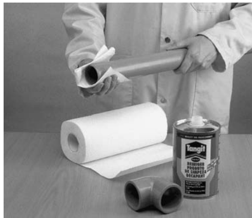
Cleaning the pipe and socket
