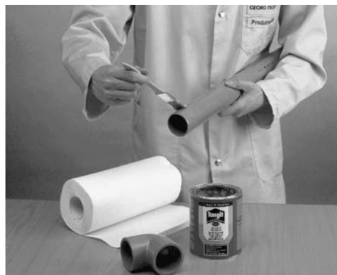
Applying the cement
