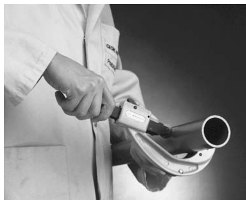
Cutting the pipe to length
